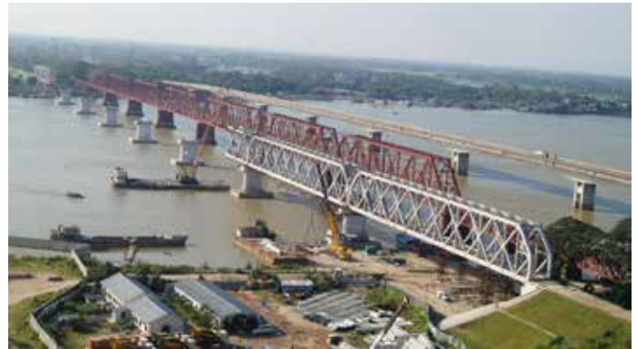
Superstructure Construction - Bhairab Railway Bridge, Bangladesh
