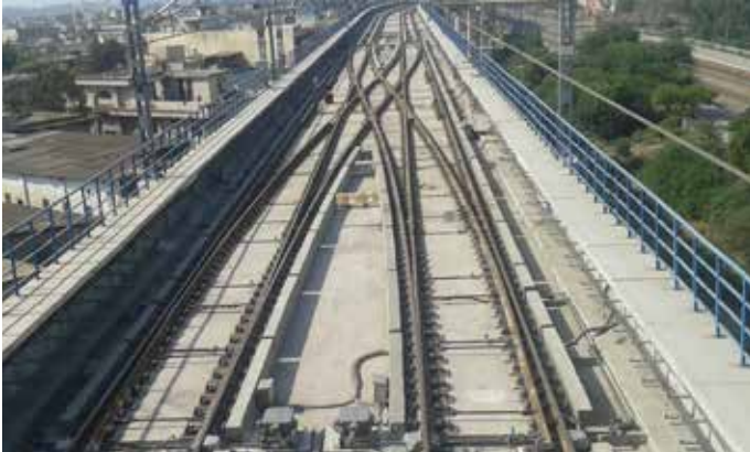
A Ballastless Track Badli of DMRC CT-4
