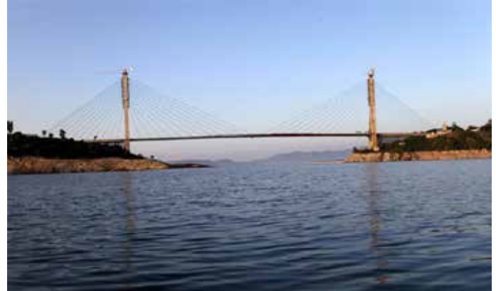
Basholi Cable-stayed Bridge in Jammu & Kashmir
